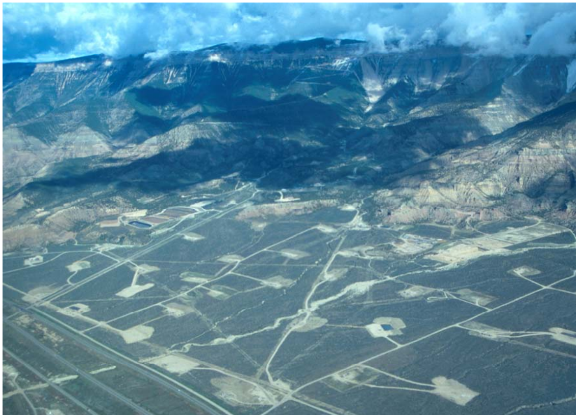
Oil well pads and infrastructure on Colorado's western slope
